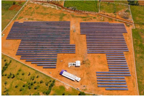
SOLAR POWER PLANT
